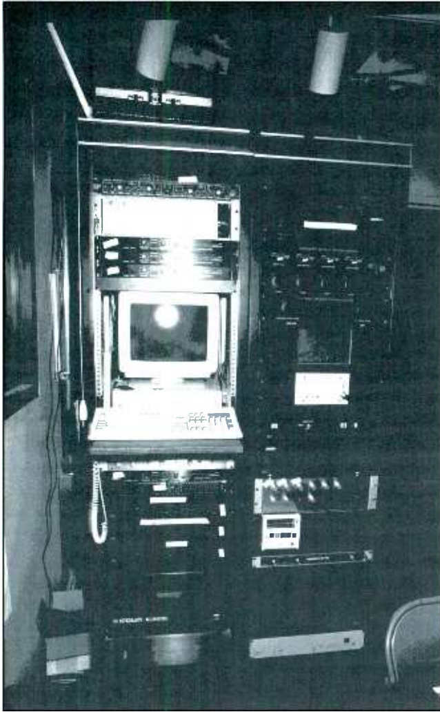
Figure 2. The Crown IQ host computer with AMX touch screen. This is located in the main sound booth at the dome.
